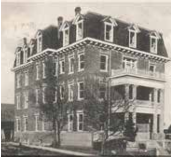
Original building, Dickson Memorial.
