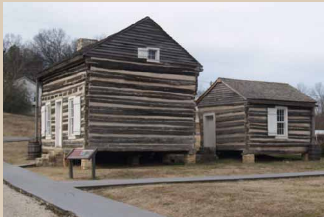
The limestone jail, above, has been used for a variety of purposes since its construction in 1873 but was restored by Arkansas State Parks in 1990. At left is the Ficklin-Imboden log house, complete with period furnishings, and below, the courtroom.
